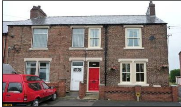
Good quality 19 th century brick terraces, but the one on the left has lost much of its character with inappropriate modern replacement windows, doors and boundary wall, while the example on the right retains the original design distinctive and valuable features.
