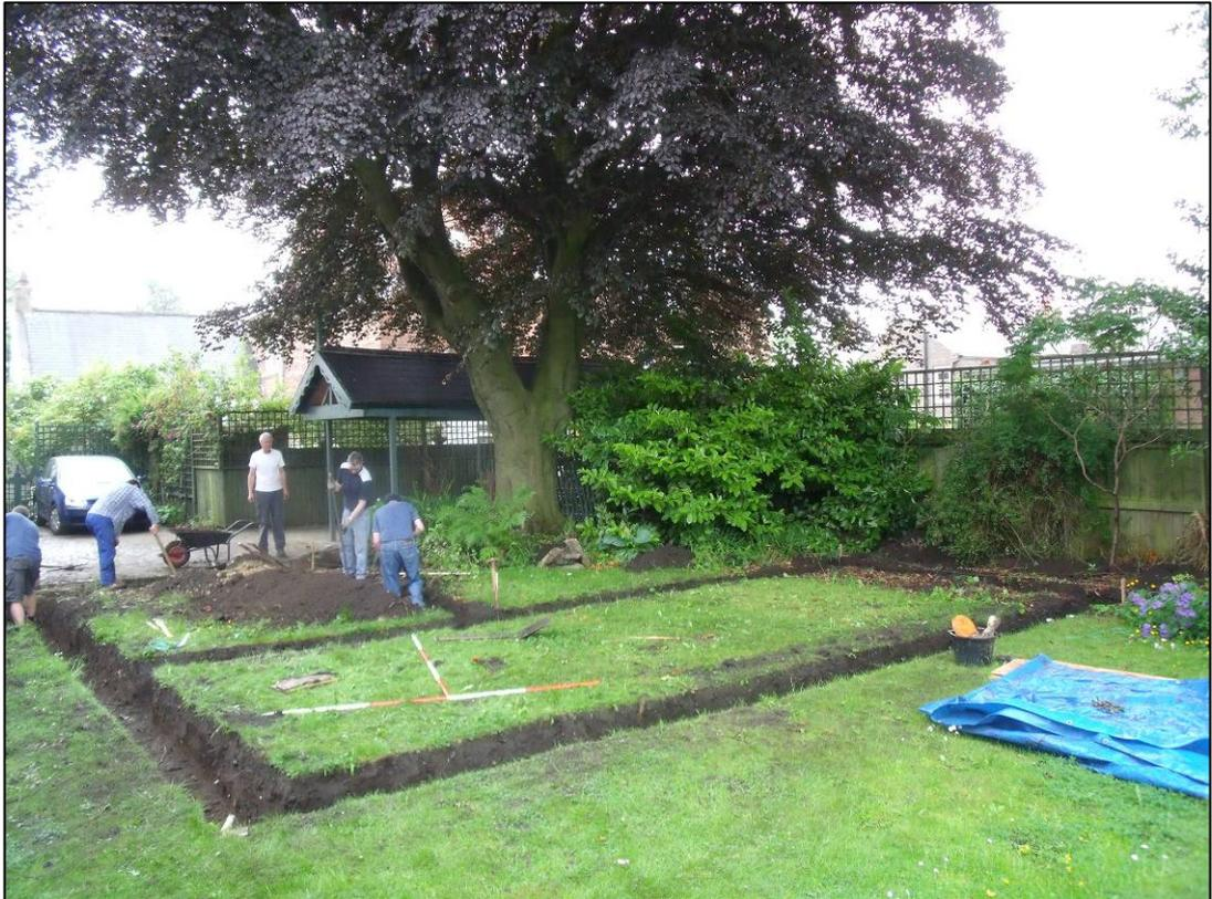
*Figure 3. Completed excavation of foundations.*
