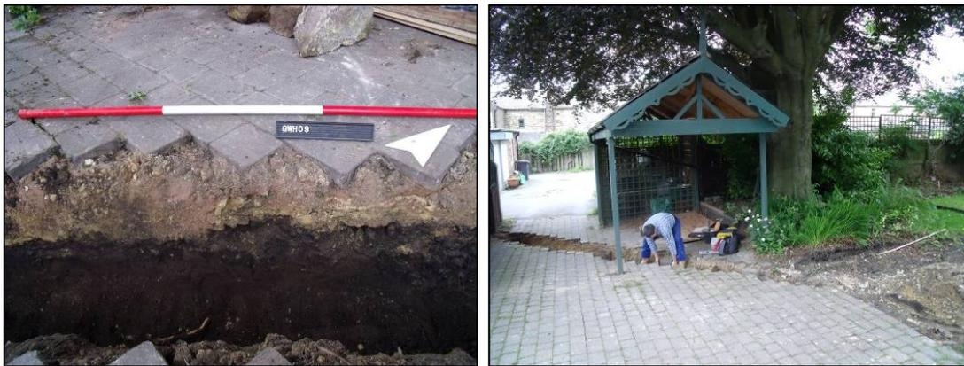
*Figure 4. Service trench running south-west from new garage-workshop to connect with existing services.*
