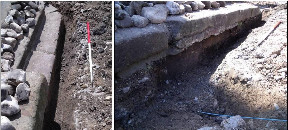
*Figure 3. Maximum depth of excavation along the west side (right), and on the north-west side where the spur trench connected to an existing electric supply.*
