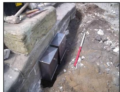
*Figure 4. North side of Butter Cross showing maximum excavation and installed metal electrical supply boxes.*
